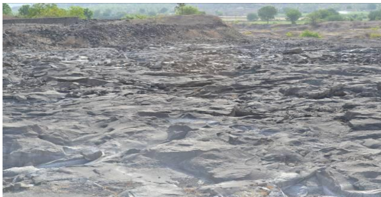
Figure 1.1 selected Photographs showing Pitching repairs, Tail channel repairs and Approach road to dam.
