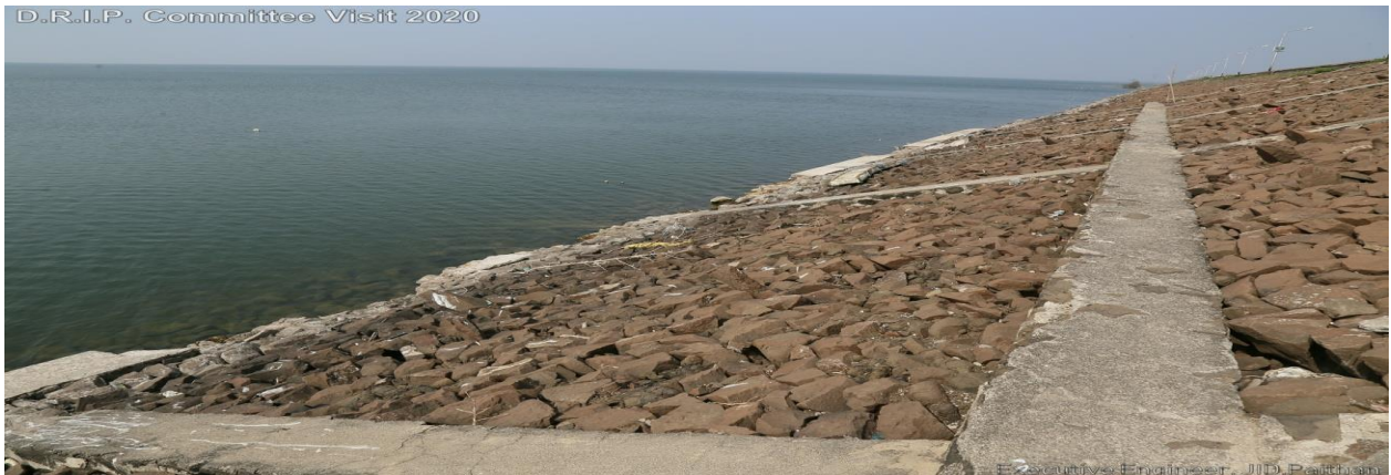
Fig 1.1 provide photographs of key infrastructure proposed for rehabilitation works.
