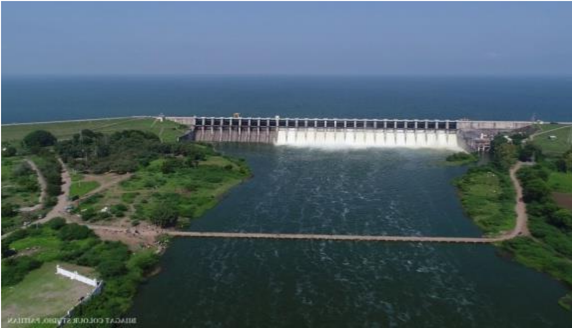
View of Dam
