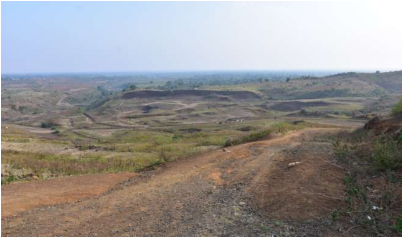
Approach Road to Dam Top
