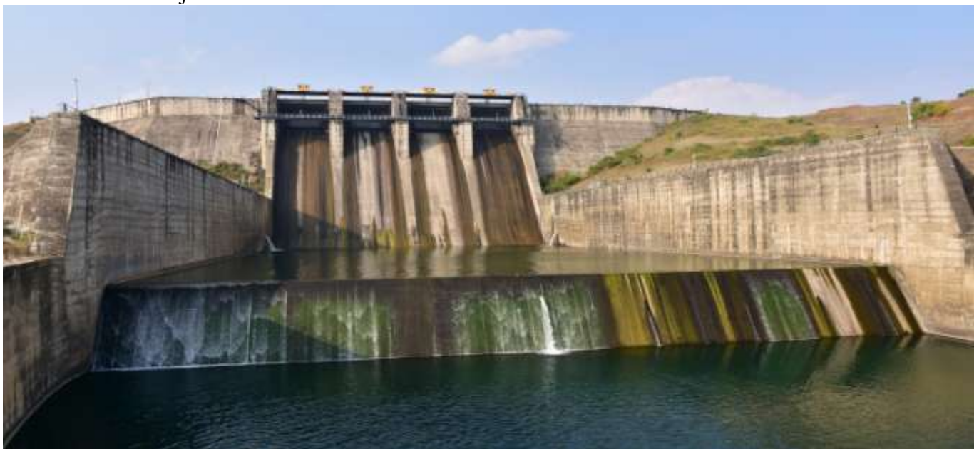
Figure 1.1: Selected Photographs of Improvement/Intervention area
