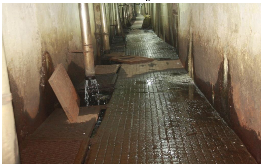
Inspection gallery cleaning of V.P.D
