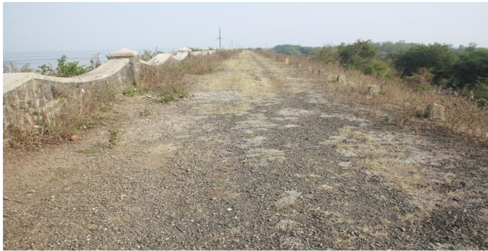
Re surfacing of road at dam top
