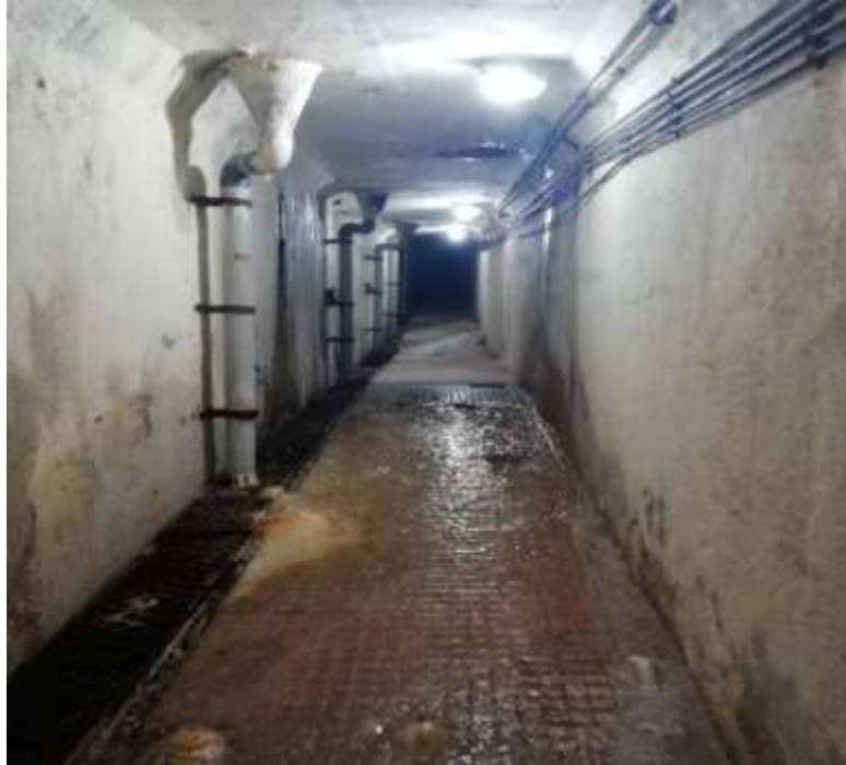
Foundation gallery VPD running full with discharge, wet gallery walls, water accumulation in gallery
