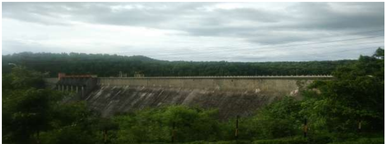
View of Dam
